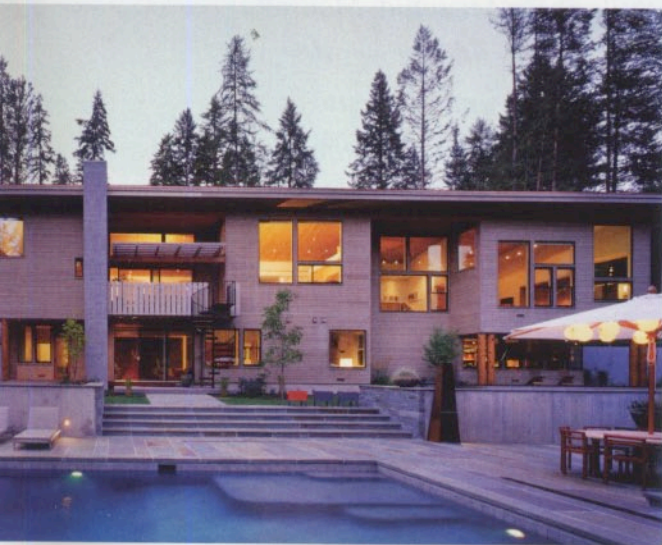
(Above) The maximum use of windows on the south side of the house gives optimum sunlight to the interior. The placement of the adjacent patio and pool allows the residents to take advantage of the sun's natural light and heat.
